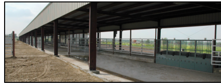
The largest individual feed intake system in the southern United States.
